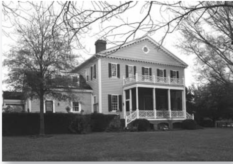
South (rear) view of Chastain
